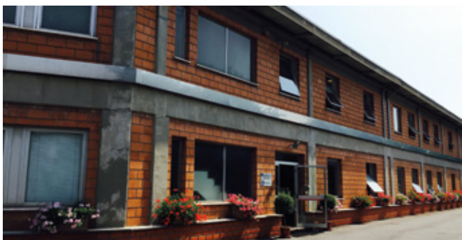
UFLEX & ULTRAFLEX - Headquarter in Busalla
