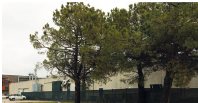
UFLEX - Factory in Tregnago
