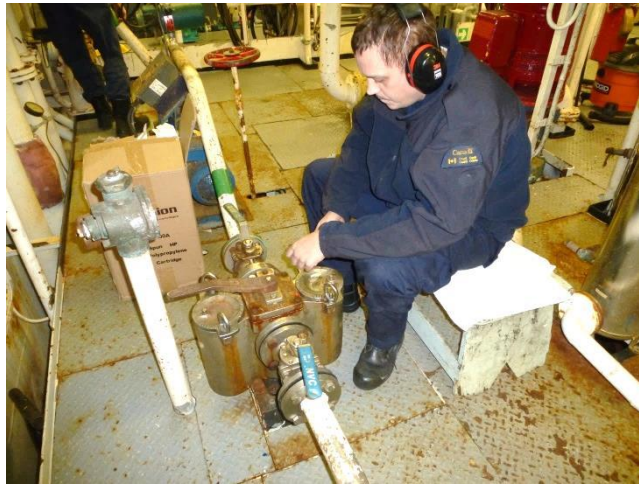
Figure 18. Seawater passes through a filter before going to the pump (in background). When the ship is in sea-ice the flow is switched from one filter to the other to allow the necessary frequent clearing out of slush from the filter. This picture is from a previous year but is the same strainer configuration for 2022.
