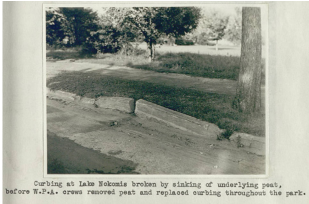
Figure 41 Broken Curbing. Curbing at Lake Nokomis was broken by the sinking of underlying peat and required WPA crews to remove the peat and replace the curbing. (Source: Minneapolis Board of Park Commissioners, 1939)
