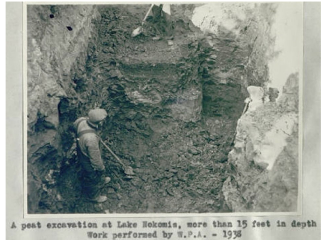
Figure 40: Peat Excavation. WPA crews excavating peat that was more than 15 feet in depth (Source: Minneapolis Board of Park Commissioners, 1938)
