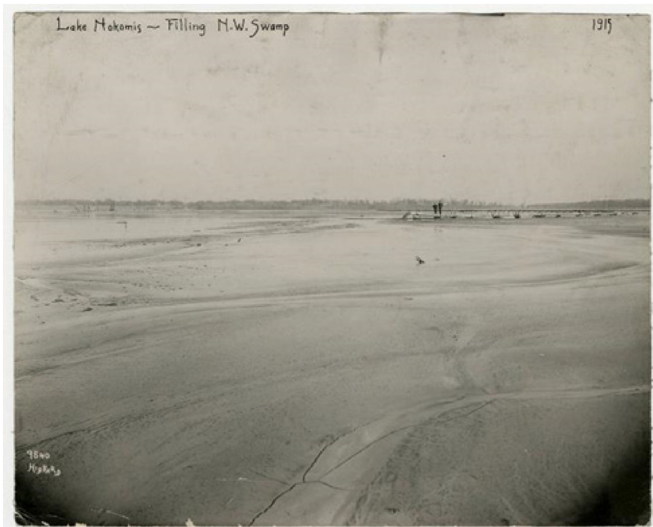
Figure 30: Filling Swamps. Dredge fills were placed over a swamp northwest of Lake Nokomis in 1915. (Credit: MPRB, 2021)
