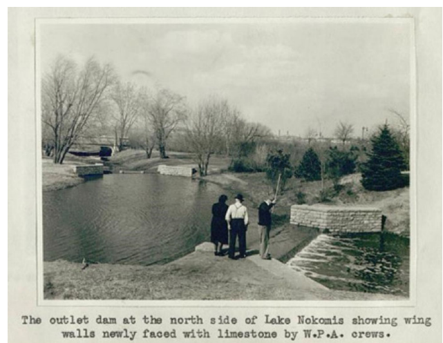
Figure 77: Lake Nokomis Outlet. Photo Caption: The outlet dam at the north side of Lake Nokomis showing wing walls newly faced with limestone by W.P.A. crews. (Credit: Minneapolis Board of Park Commissioners, 1939)
