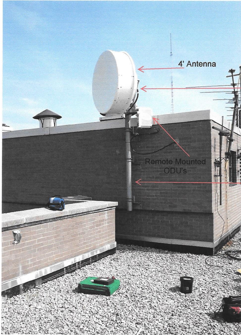
Typical Wall Mounted Antenna and ODU
