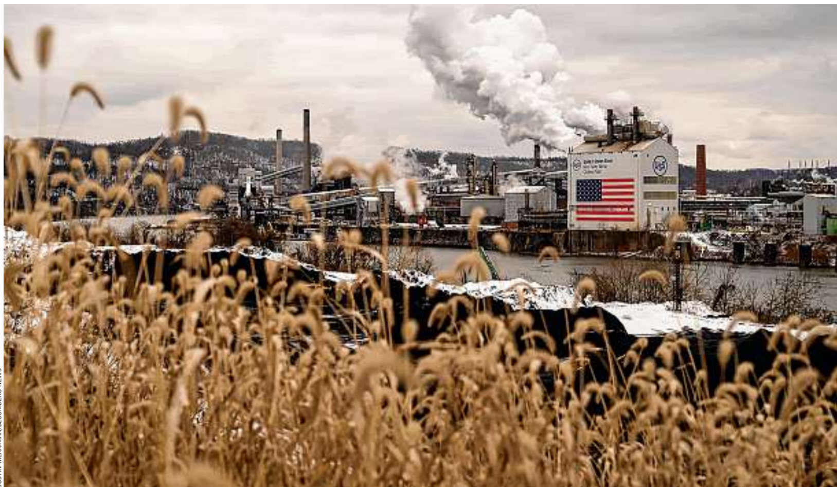
A U.S. Steel facility in Clairton, Pa. President Biden said he opposes the purchase of the company by Nippon Steel.
