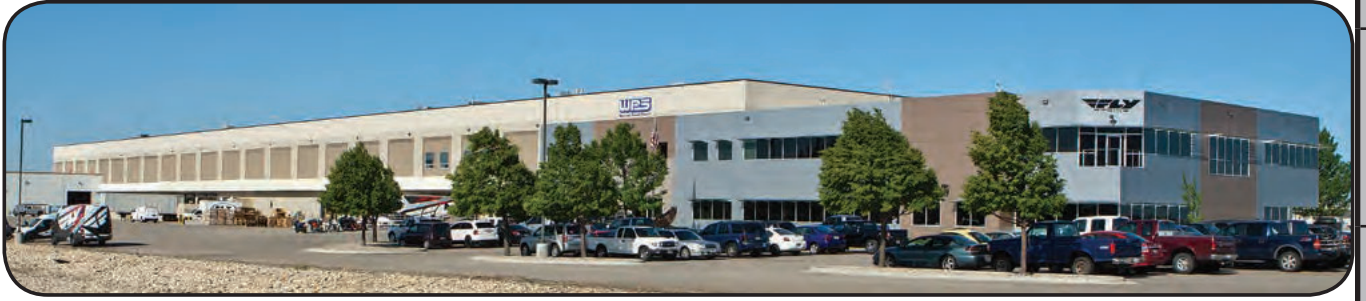
Boise, ID Corporate Headquarters and Warehouse facility 258,000 sq. ft.
