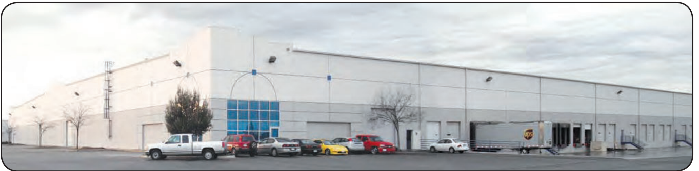
Fresno, CA Warehouse facility; 100,000 sq. ft.
