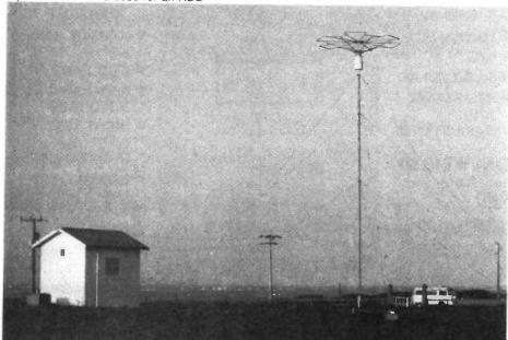
Between the very low end of the usable radio spectrum and the bottom end of the long wave broadcast band at 150KHz there are several stations designed for worldwide communications with submarines. It is only these low frequency signals that can penetrate sea water to any depth at all.
