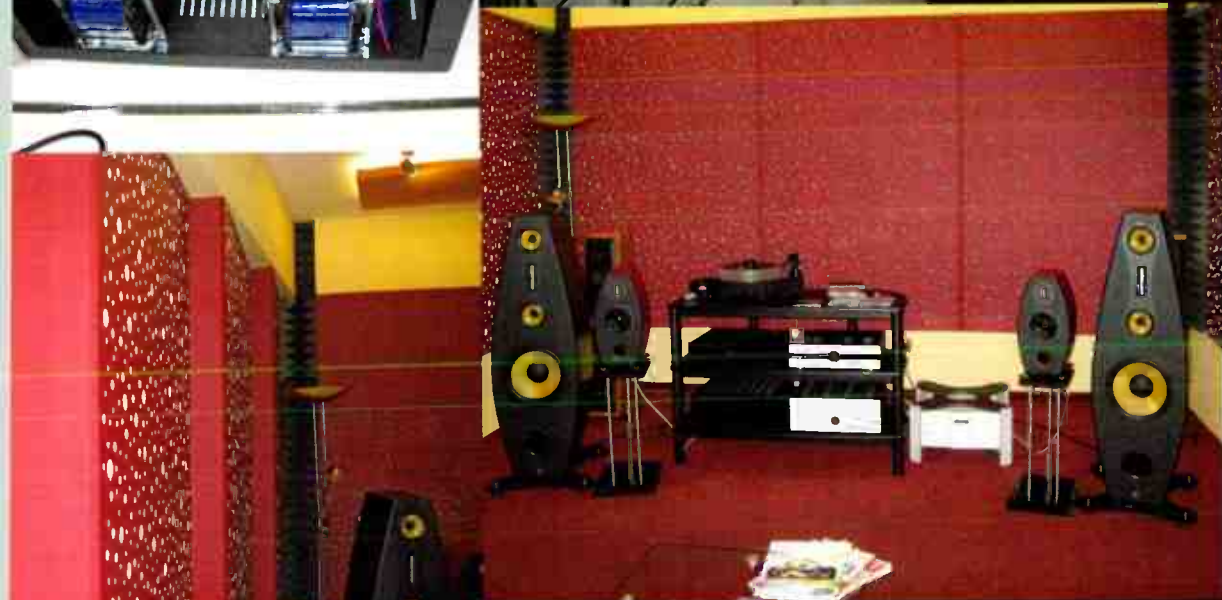
◀ The walls of the listening room are stepped in three places along the sides, and are covered with painted plasterboard that has had varying size holes drilled through it in a random order to help eliminate room resonances. The ceiling has also received acoustic treatment.
