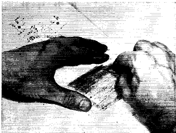
Fig. 2—Prepare the drawing for tracing by rubbing the back with the flat side of a soft pencil. Carbon paper may be used instead.
