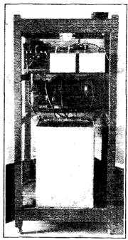
WSARO'S POWER SUPPLY UNIT The mercury are is in the tank at the bottom of the frame. Above it are to be seen the keepalive transformer, the high-voltage transformer. the filter condensers and the two chakes
