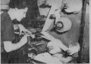
Operator of the winding machine is Mrs. Maureen McCormick, an employee of the Telegraph Condenser Company of Toronto. She is shown winding electrolytic capacitors, a highly skilled operation.
