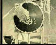
"We have had up to four inches of ice on the radome with practically no reduction of antenna effectiveness. During high winds, radome reduces pressure on the dish. (AM-TV Station)
