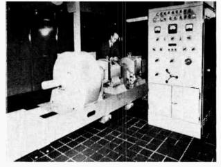
A New Brunswick Telephone Company craftsman performs a routine on an Austinlite 20 kw motor fly-wheel alternator unit, one of two such units in service with the company.
