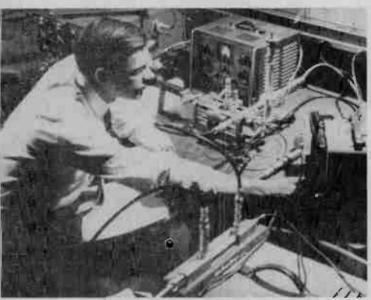
Low-noise parametric amplifier developed by General Electric Company was combined with an 18-foot high-gain parabolic antenna to receive signals from Pioneer IV more than 410,000 miles from earth.
