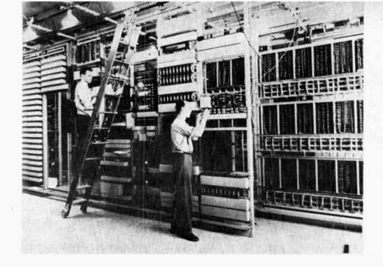
The above photograph shows typical ranks of SATT (Strowger Automatic Toll Ticketing) equipment installed in the Penticton. B.C., Toll Center of the Okanagan Telephone Company. Similar equipment is also to be installed in the Toll Center offices at Kelowna. Vernon and Salmon (Photograph courtesy Redivo Camera Centre & Studio Penticton, B.C.)
