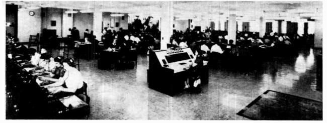
The long distance room in the B.C. Telephone Company's Vancouver headquarters buildings, showing most of the 192-position cordless switchboard. The board went into service in 1959, making it possible for operators to ring any one of some 50 million telephones in North America, without the intervention of operators at the called points.
