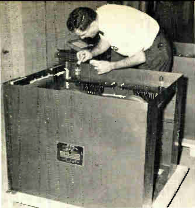
Fig. 6: This magnetic amplifier reactor assembly has no moving parts—no tubes. For motor speed control of 200 hp motors, it is rated at 173 kva, 240 v, 60 CPS.
