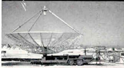
60-foot ground mounted tropospheric antenna. It's an offset paraboloid design, is fabricated of galvanized steel, and features maximum interchangeability and standardization of the various members.
