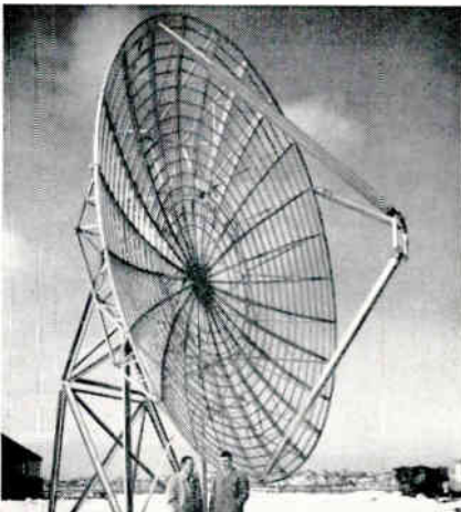
This is a 30-foot, mesh surface paraboloid (Model 101) which was designed for wide use in the fields of radio astronomy, tropospheric scatter propagation, tracking, and experimental test installations. The mount was also designed by ASI, and features azimuth and elevation adjustments at the foot plates where they can be easily reached.
