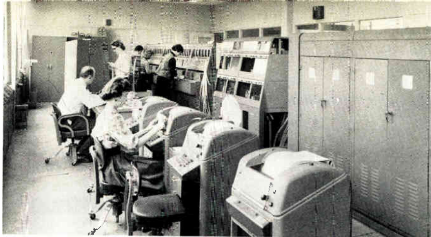
FFig. 1: Univac, with its 5,400 heat-generating tubes, requires extensive cooling equipment.
