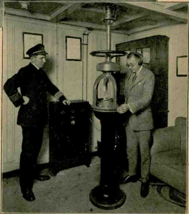
Dr. Kolster, inventor of the modern radio compass, operating the instrument on the S. S. "Leviathan." Above, loop with its supports on the flying-deck of the "Leviathan"; below, close to ceiling, the capacity compensating device, next, hand-wheel for rotating loop, mechanical compensator for error, sight-wires, dial; to the right, the six-tube receiver.
