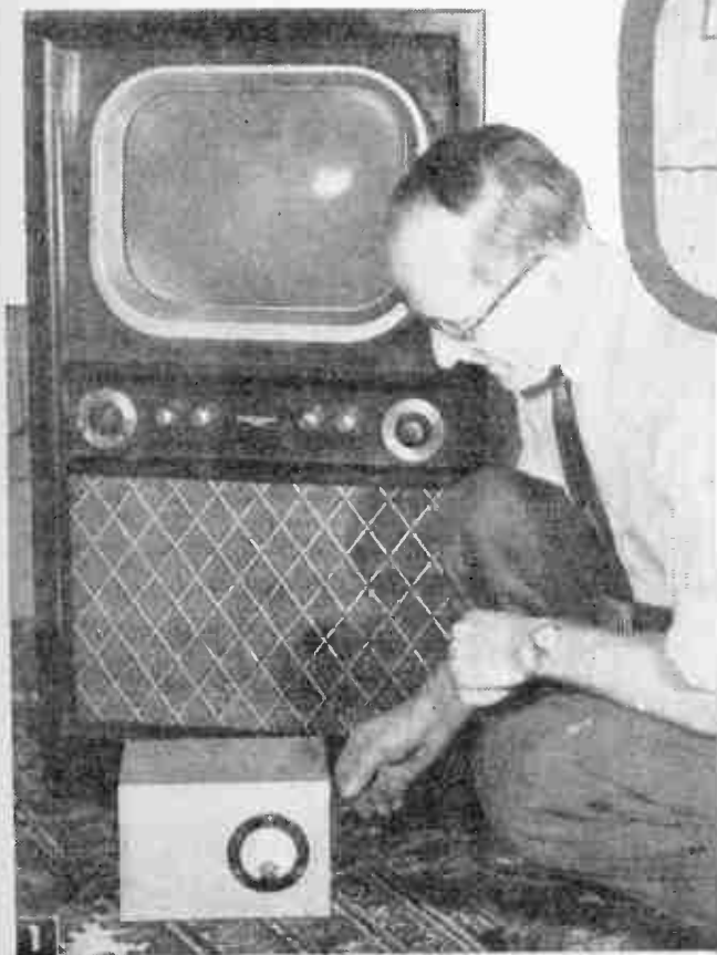
Picture wouldn't fill out screen when set was operating on 106 volts (A). Increased brilliance and full screen (B) improve picture after boosting line voltage to 112-115 volts.
