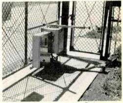
Fig. 5 Motorized gate controllers: Their Installation involves excavation and laying underground cable.
