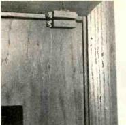
Residential security devices can encompass such simple items as magnetic sensors mounted on doors or windows which sound an alarm if a break in occurs to such sophisticated products as the seismic detector system, at left, by Intrusion Detection Systems which is designed for both industrial and upper income home protection.
