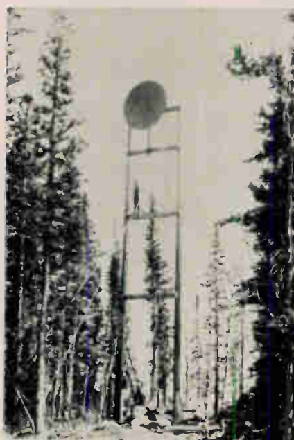
A 90ft tower carries a 10ft dia parabolic antenna which is used at Escalante, Utah, to bring in educational TV programs. The mast is constructed from two trees. Several TV translators are attached near the tower.
