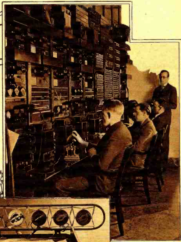
THE CONTROL ROOM. (Below, left.) These amplifiers under the steps of the Capitol, strengthened the speech and music before they reached the telephone exchange. © Kadel & Herbert.
