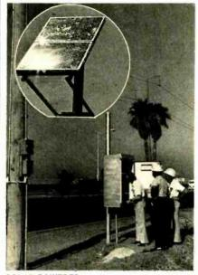
SOLAR-POWERED traffic counter being tested in Glendale, AZ. Inset shows solar silicon array.
