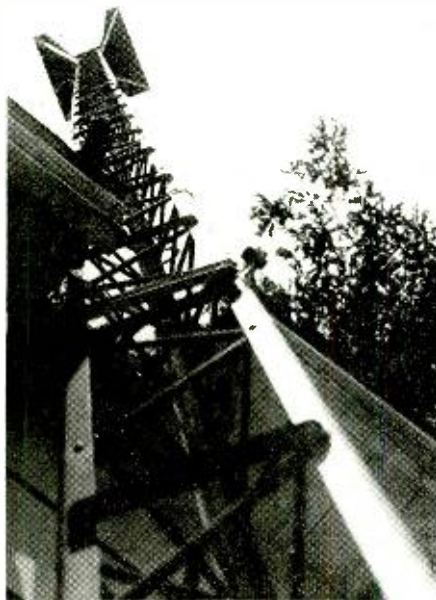
Fig. 6—Looking up along tower will tell you whether or not it's straight.
