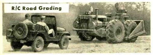
Push-button construction work is on the way. A standard U.S. Army "Tournadozer" equipped with standard military radio equipment (above) can be put through its paces by helicopter or jeep with transmitter and special control box up to a distance of 15 miles. It's under test at Fort Belvoir, Va. POPULAR ELECTRONICS
