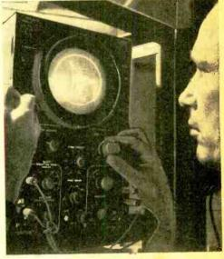
Answers to trigonometric problems are furnished by series of dots on ascilloscope.
