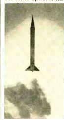
physical characteristics of the ionosphere, gathering information on how radio waves are transmitted. During its trip it took photos and conducted many experiments —with no human being on board. Made by MartinAircraft of Baltimore, Md., this rocket reached a speed of about 4100 miles an hour. It weighs  $7\frac{1}{2}$  tons and is 45 feet long.
