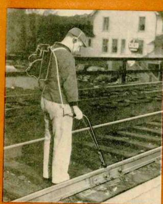
Using a portable ultrasonic flaw detector to check a railroad track rail for detects or cracks.
