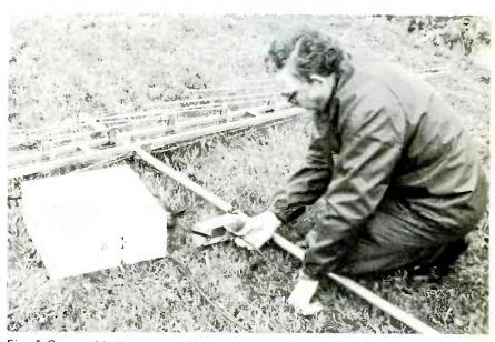
Fig. 5 Coax cable is not sensitive to metal near it, so standoffs are not necessary. However, the coax should be secured, perhaps by layers of plastic tape, to the mast and the tower, thus preventing it from being moved by the wind.
