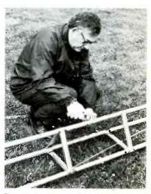
Fig. 2 Various sections of the tower should be assembled on the ground.
