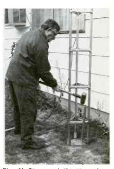
Fig. 11 To prevent the tower from tipping, the base plate is firmly secured by three base stubs, which are driven into the ground.
