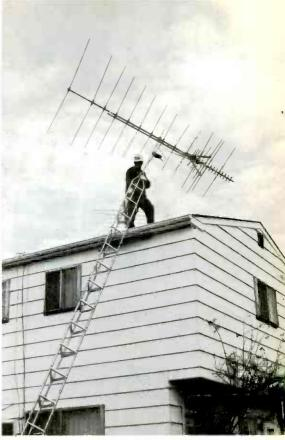
Fig. 8 The man on the roof lifted the assembled mast and antenna, connected a safety rope to prevent it from falling accidentally, and both men positioned the tower approximately where it should go.
