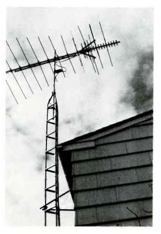
In fringe reception areas, you have to work hard for every microvolt of TV signal. Three things are essential: the antenna must have very high gain; a low-noise mastmounted preamplifier is needed; and, the antenna should be mounted up high.
