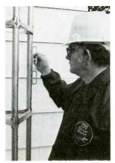
Fig. 10 Gentle taps of a sledge hammer moved the bottom of the tower to provide true vertical, as measured with a level.
