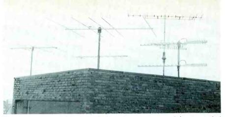
Six antennas, many of them single-channel yagis, were used for one typical MATV installation in a large apartment building.
