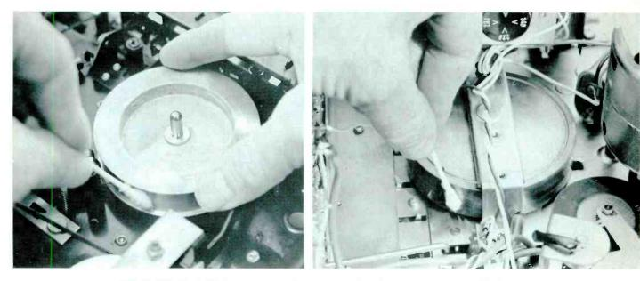
Step 8. The flywheel in most recorders also requires frequent swabbing off. Its drive surface collects grime and evaporated-oil residue. Clean the outer rim and the shaft with alcohol. Repeat the swabbing several times until a clean cloth or Q-Tip shows no trace of dirt.
