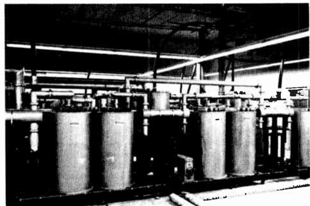
Figure 15. This Senior Road, Houston, Texas ten-port diplexing system, combines nine FM stations into one community antenna. It is capable of 350 kW total input power. (Courtesy Harris Corp.)
