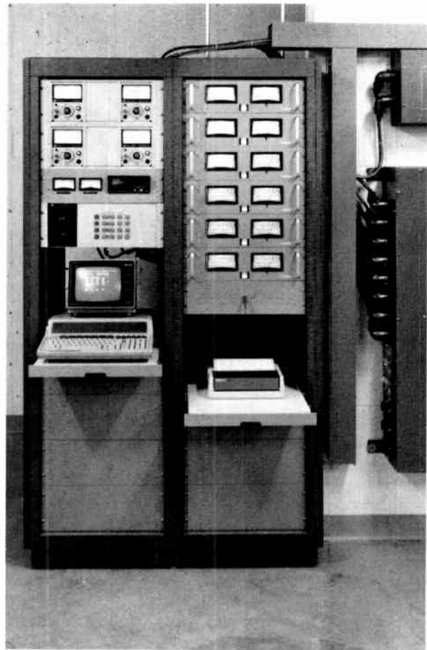
Figure 46. RF monitor and control system in St. Louis. (Courtesy of EZ Communications, Inc.)
