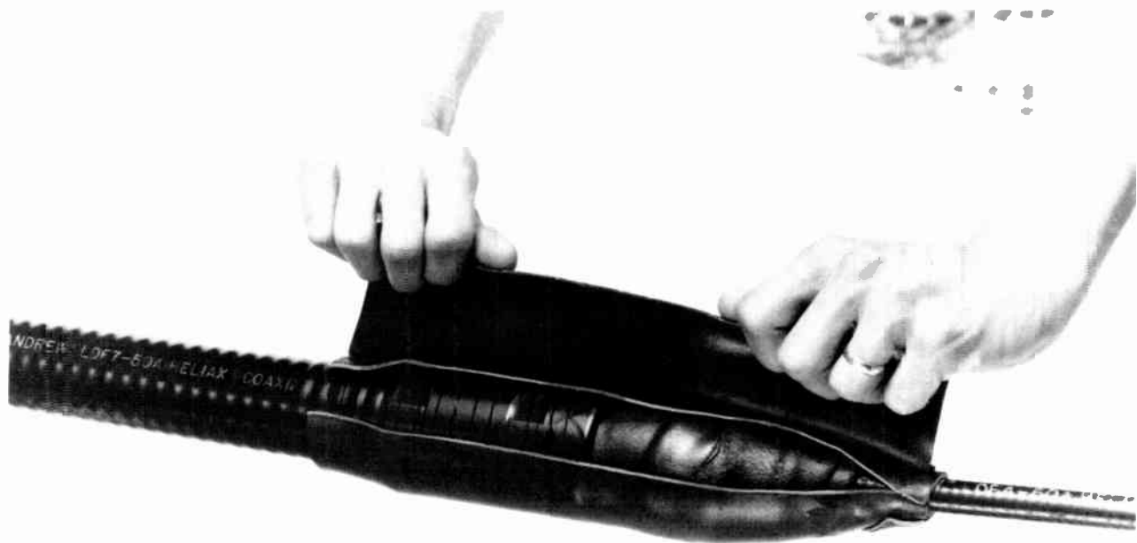
Figure 12. Cut butyl rubber tape into six 12" lengths. Form a tapered surface by starting with two tapes folded to half their widths. Finish with one full-width tape.
