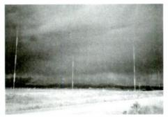
WWVB transmits a time signal on 60 kHz
