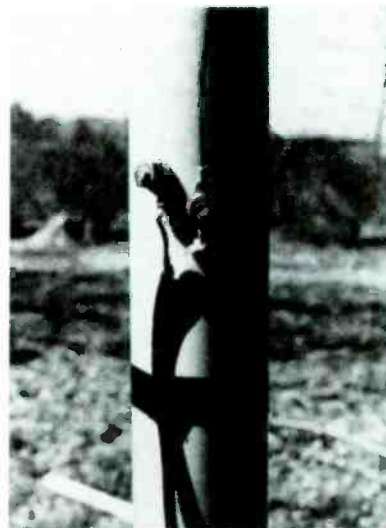
Fig. 5—Coax lead-in cable should have its shield connected to a dummy terminal that provides good mechanical support for the cable and keeps the weight off the solid inner conductor.
