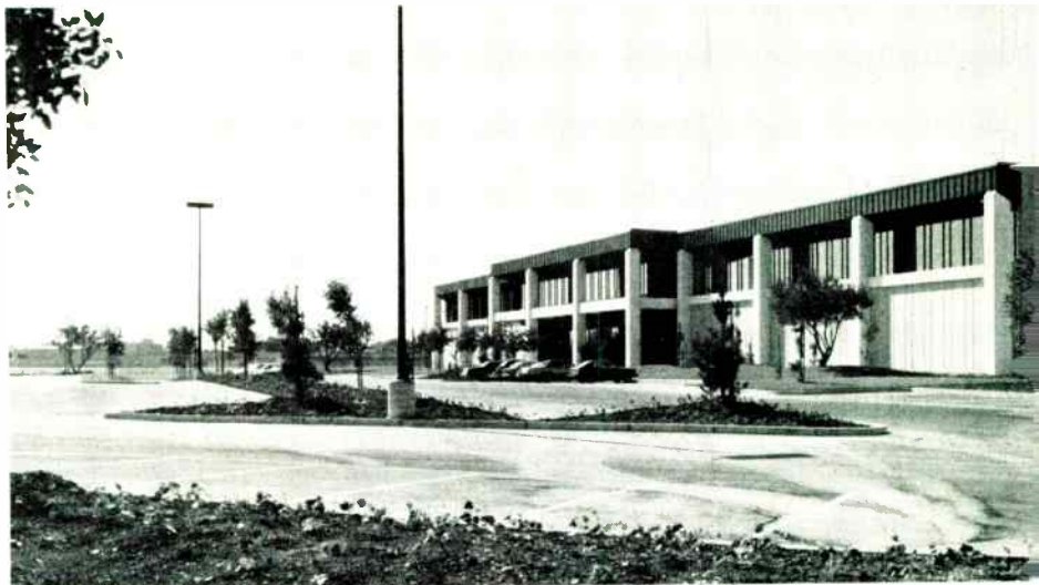
Headquarters. This is Advanced Micro Devices Inc. in Sunnyvale, Calif. The company has decided it won't need a bipolar facility scheduled to go into half of another building in nearby Santa Clara.
