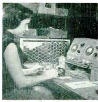
Jig on bench speeds testing of plug-in electrolytics for leakage
