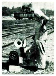
Maintaining freight-yard communications; whí radio in switch engine features failsafe operation. Talk-back loudspeakers keep yard workmen in touch
