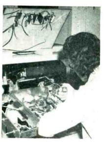
Inspection position on chain-conveyor assembly line, showing method of mounting layout print. All parts and leads assigned to this operator have been mounted on this print in their correct positions
