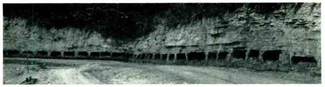
Appearance of hillside after coal vein has been mined by machine. Three-foot ribs are left between 116-inch-wide cuts to hold up hill. In present operation, holes go in only 690 feet because additional conveyors are not yet available
