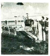
Microphone lowered into tank picks up high frequency sounds emitted by porpoise
