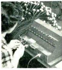
Operator matches corresponding pairs of conductors with this test set to check for short-circuits in cables at final electrical inspection station
