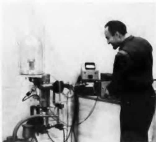
Vacuum system used in depositing sub-micron-thick dielectric films on various substrates at Nuclear Research Associates contains plasma that aids a gas-phase reaction. The dark plates in the Bell jar are electrodes, on which the deposit is forming. The reaction is being controlled here by Jerry Goldman, vice president and research director of the company.
