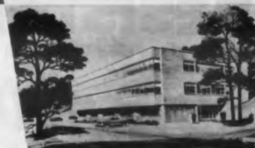
Latest GPL engineering building, for which ground was broken recently. ▶
