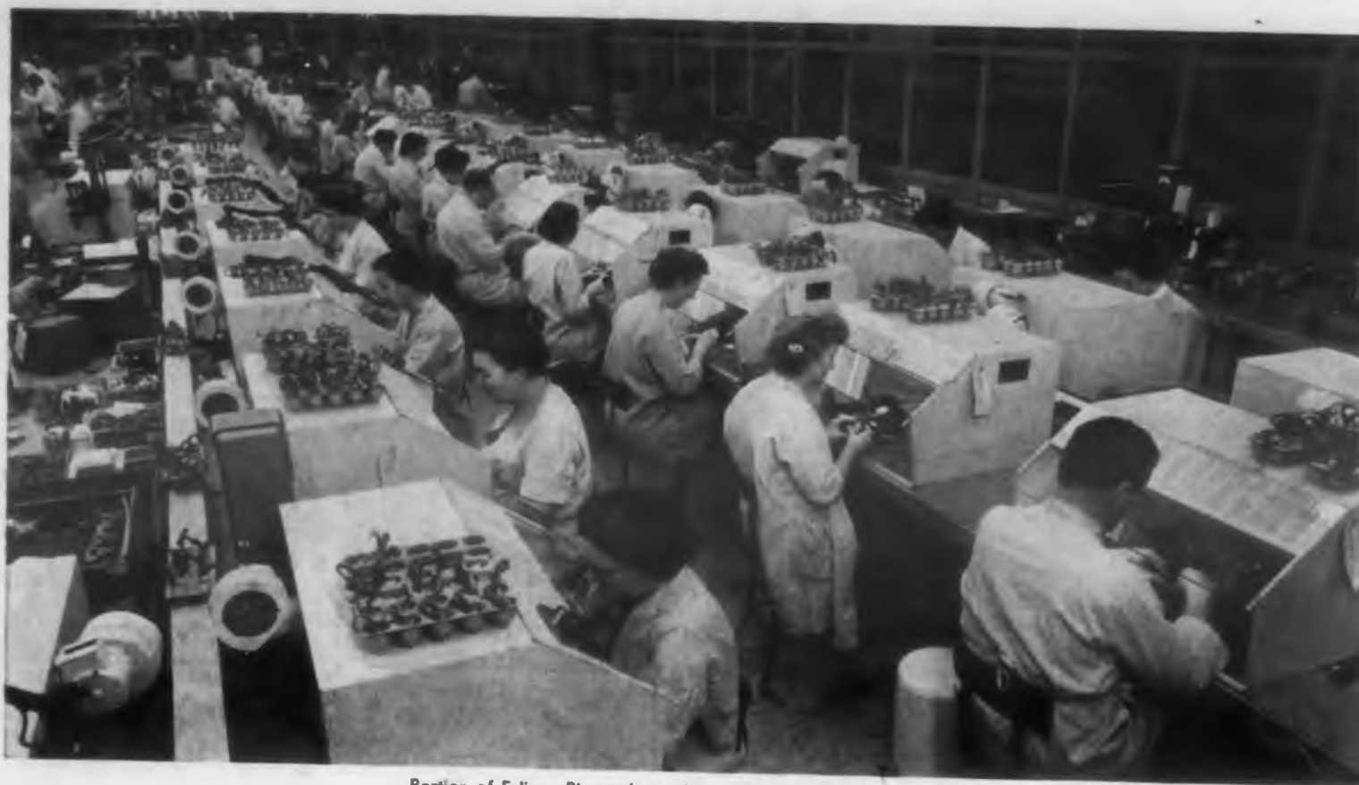
Portion of Eclipse-Pioneer's synchro calibration and test facility.
