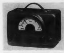
The A.F. Oscillator 816 gives an output from 30 cps to 30 kc in three ranges. It is intended for adjustment of af amplifiers in PA work and af stages in radio.
