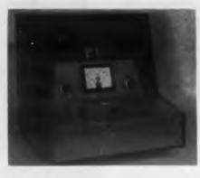
This portable leak detector is capable of exacting tests either evacuated or pressurized systems. Known as Type 24-210, it can be used to show the existence or absence
