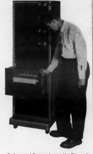
Rack-mounted Dynograph assembly. The amplifiers are at the left, the input couplers to the right. The stylus control panel is below, and just above the slide-out recorder.
