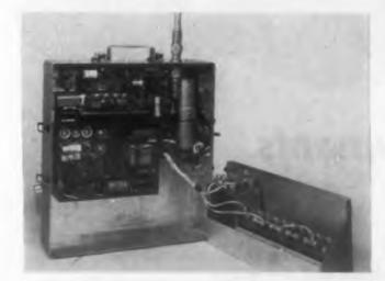
The silver cell batteries contained in the 15 pound pack operate the equipment for 5 hours and can be recharged.
