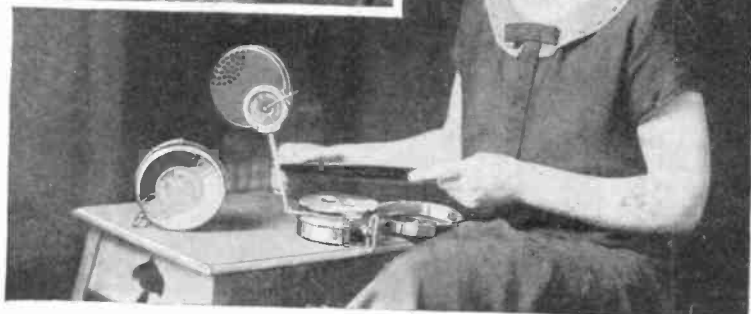
The young lady at the right is showing you how to change a record on the new baby phonograph. The complete mechanism folds up into the unit shown above.
