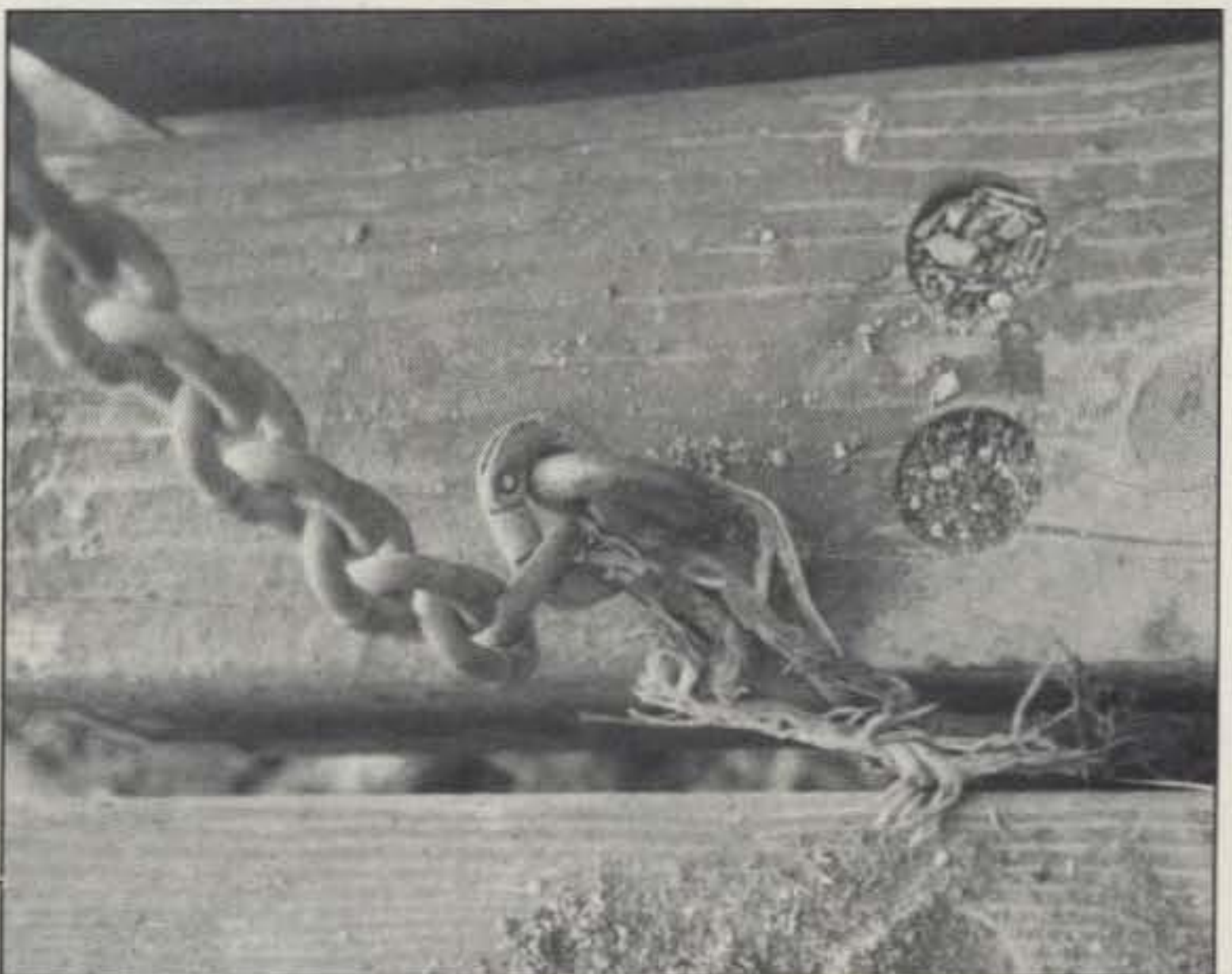
Photo E. Several hunters walked right over this antenna connection. A corroded piece of wire ties the transmitter under the ramp to the chain/antenna. Can you see it?
