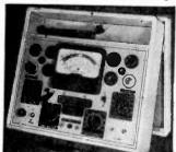
Tube Tester has speedy leak-age-short tests between all elements. Separate noise test for tubes that otherwise test "good". Large scale 4 1/4" "good". Large scale 4½"
