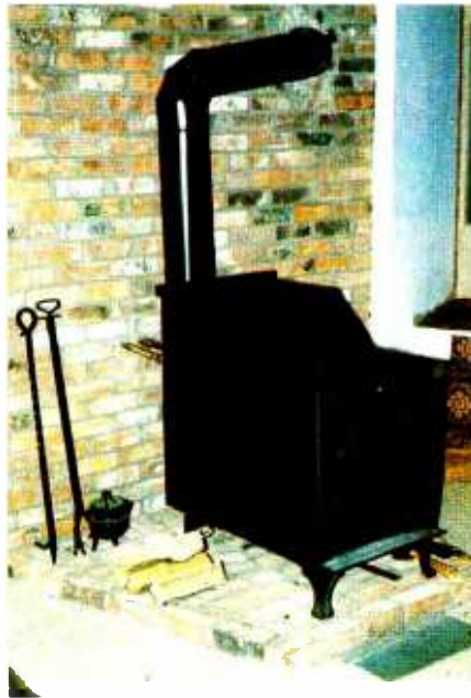
Photo 1: The Hydrostove is installed in the corner of the Circuit Cellar. Take note of the two copper pipes coming out the rear of the stove into the wall. The pipes, which are buried behind the wall and above the ceiling, go to the furnace, which is 35 feet away.
