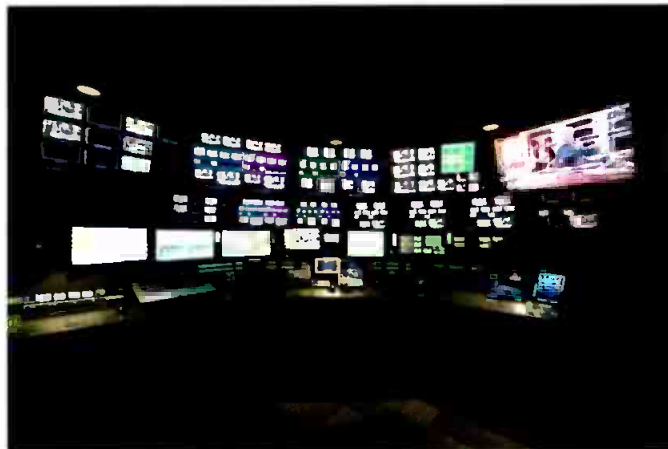
In the newly redesigned control room, Evertz monitors route the appropriate multiviewer outputs to one of 13 overhead displays, which are fed by a redundant analog Raritan KVM matrix.
