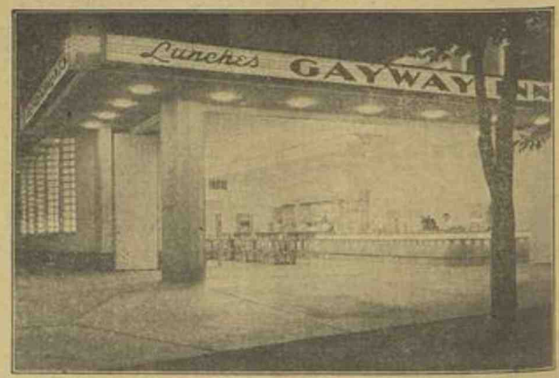
OPENED DURING THE 1935 SEASON in Lakeside Park, Denver, the $25,000 Gayway Inn is called one of the beauty spots of the 160-acre park. Constructed with open front equipped with sliding doors, the structure is of modernistic design, featuring use of glass brick, fluorescent lighting and terrazzo decorative floor. Booths and tables of solid maple match serving table decorations. Stainless steel equipment is used thruout fountains and serving tables.
