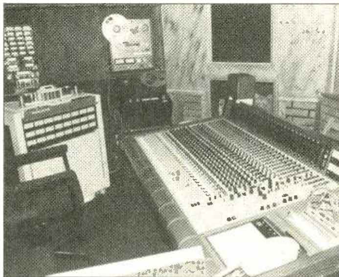
Control room with MCI 428B console and Otari MTR-90
