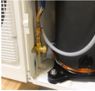
Figure 22: Liquid line service port
