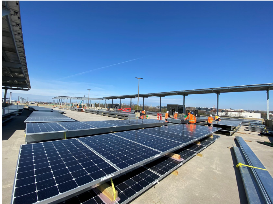
Solar Installation at Anacostia Garage
