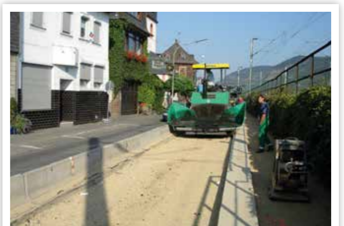
PAVEMENT REHABILITATION ON MUNICIPAL ROADS
