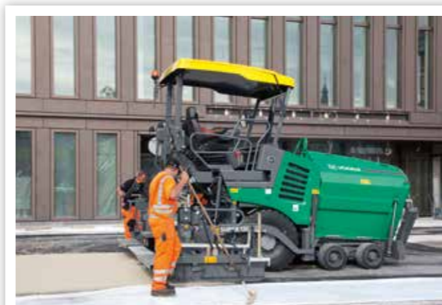
ASPHALT PAVING ON COMMERCIAL SITES
