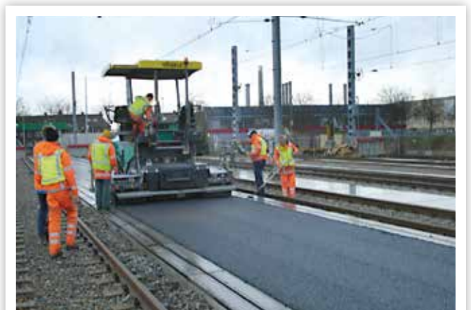
ASPHALT PAVING ON RAILWAY PLATFORMS
