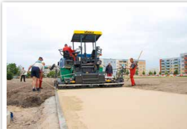
PAVEMENT REHABILITATION ON ACCESS ROADS
