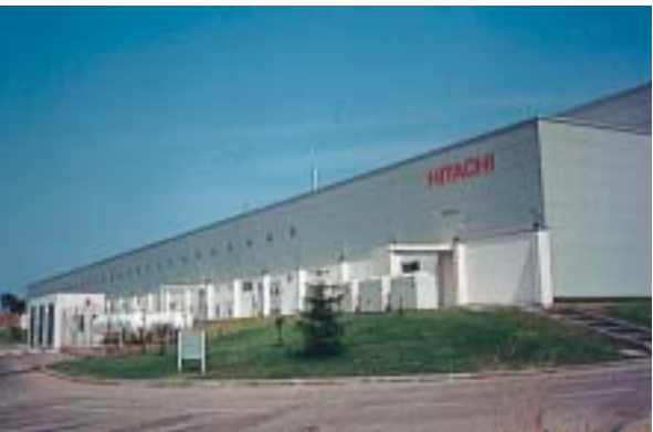
Hitachi Air Conditioning Products Europe (HAPE works, Spain)
