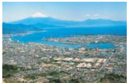
Hitachi Air Conditioning Systems Co., Ltd. (Shimizu works, Japan)
