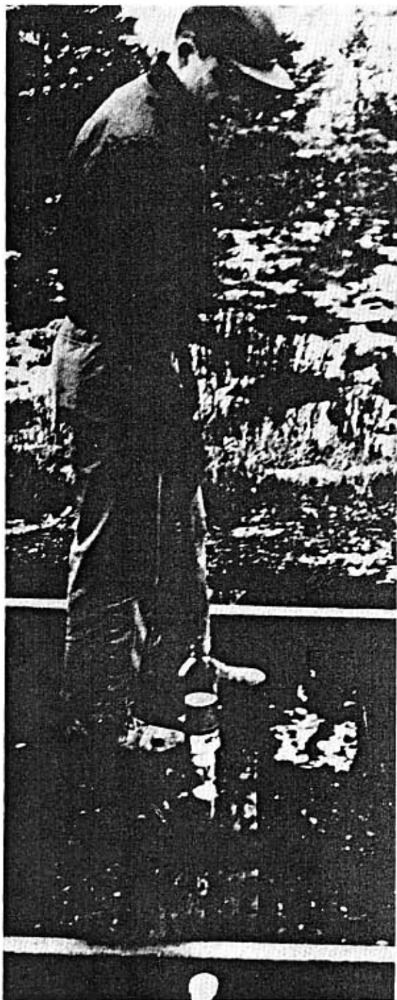
Figure 3-20. Spot marking ties for removal.
