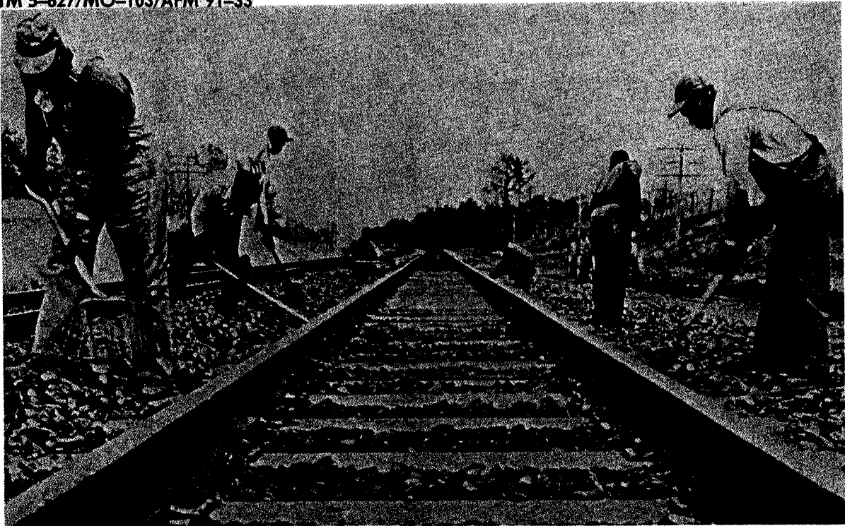
Figure 3-6. Hand-placing ballast after mechanical distribution.
