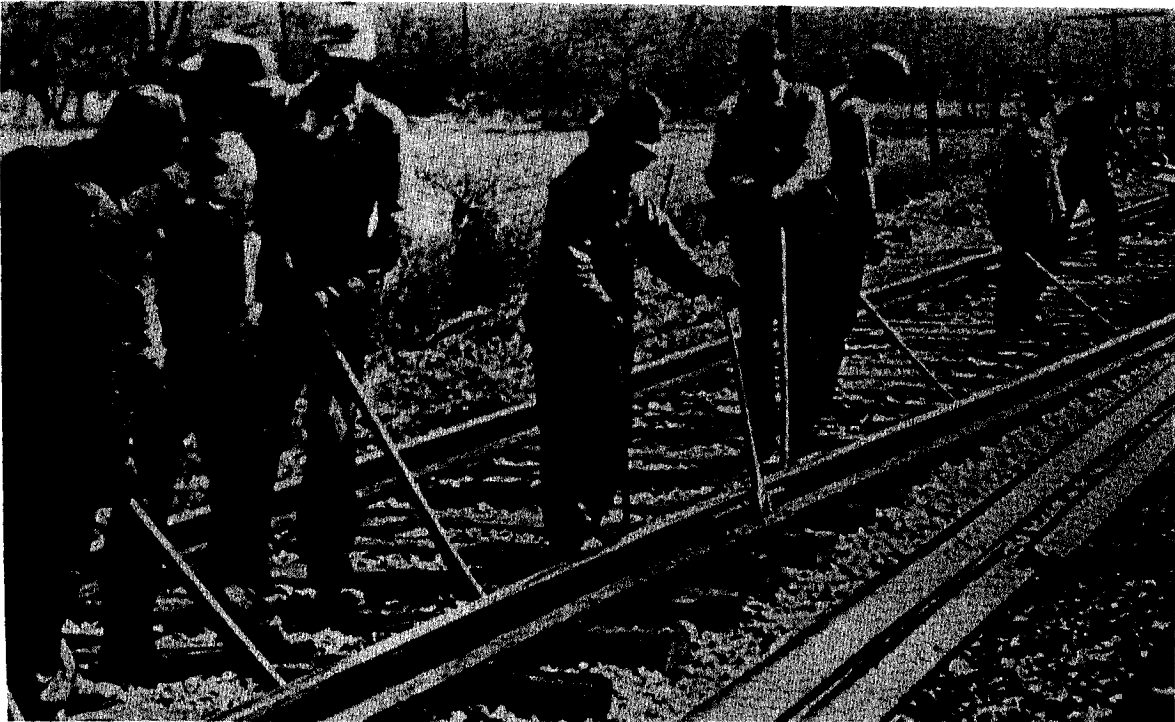
Figure 3-36. Rail being lined out.
