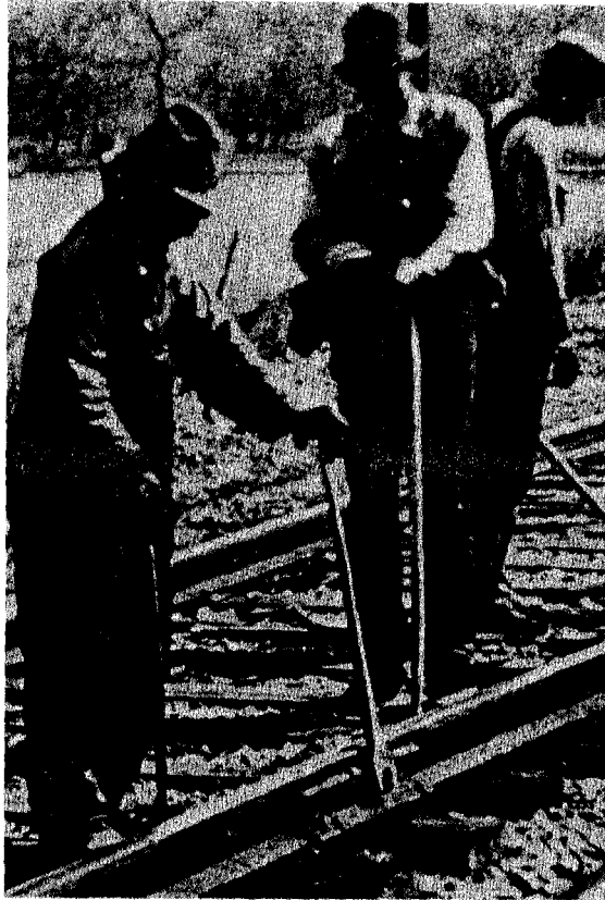
Figure 3-44. Using a hand wrench.
