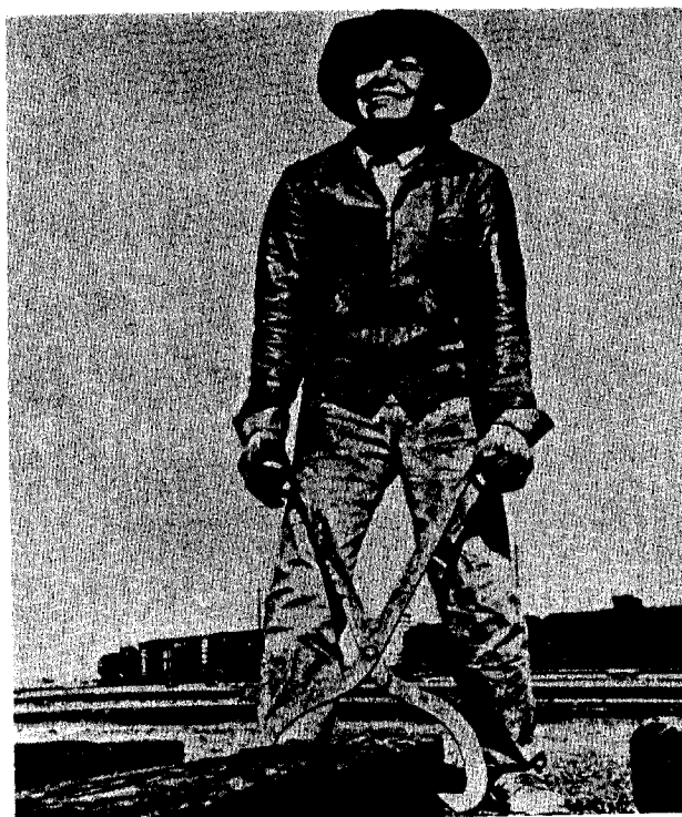
Figure 3-16. Handling treated wood ties.
