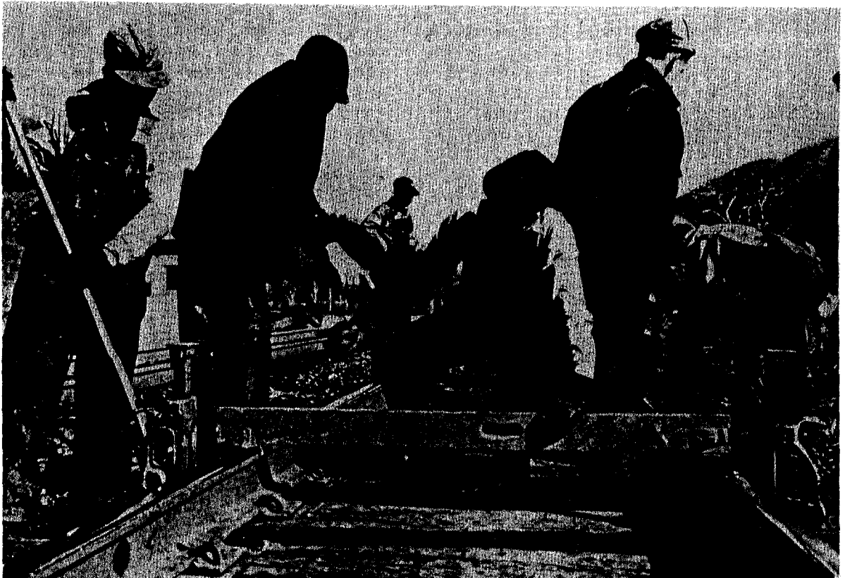
Figure 4-3. Surfacing track with a leveling beam.
