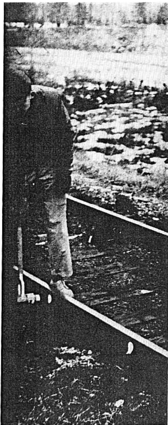
Figure 3-21. Spot marking rail with paint.
