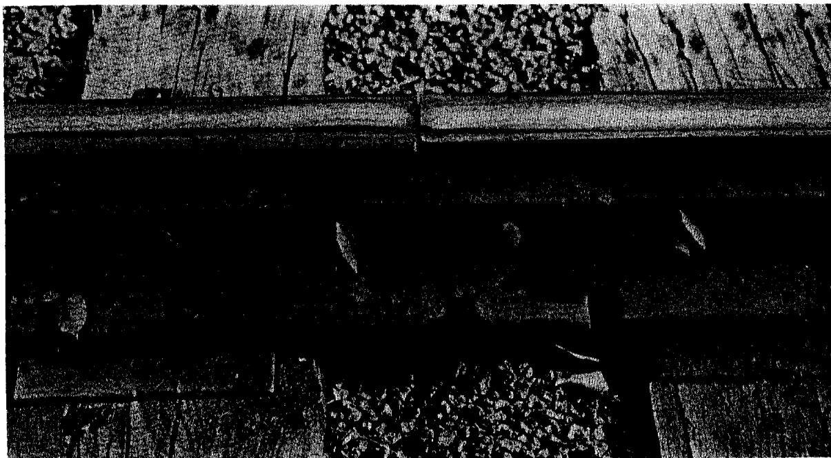
Figure 3-43. Joint-bar installation.
