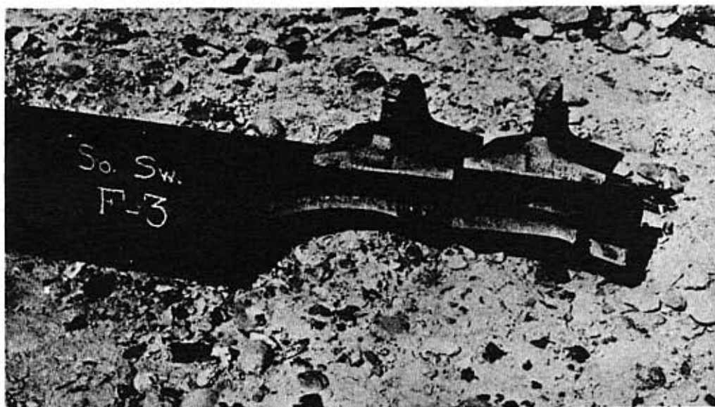
Figure 3-30. Broken base and web.
