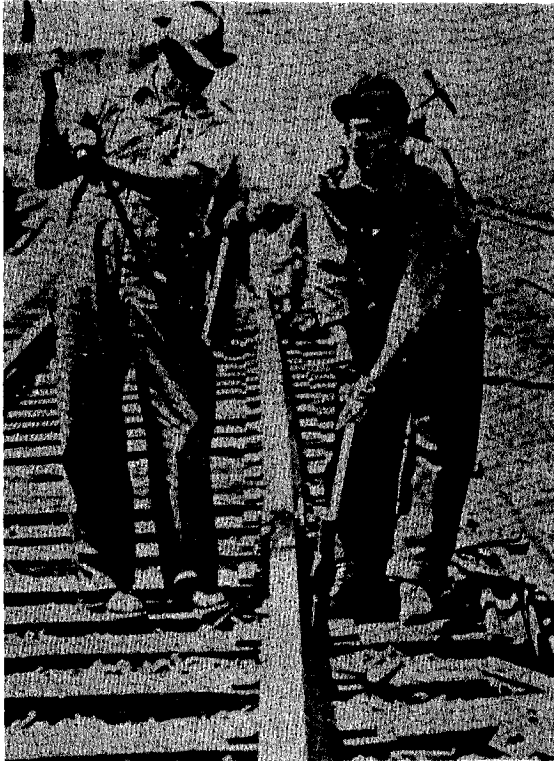
Figure 3-38. Driving spikes with a spike maul.
