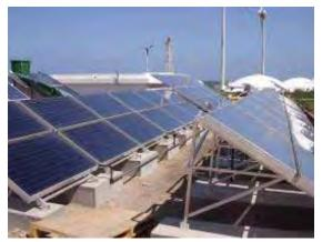
Figure 2.10. Flat plate collectors on mounting construction.
