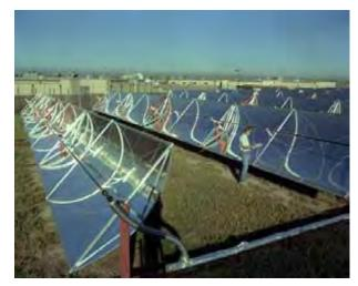
Figure 3.17. Parabolic trough collectors used to heat water at a large prison facility in Colorado.
