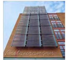
Figure 5.4. Collectors integrated into the façade as a structural element.
