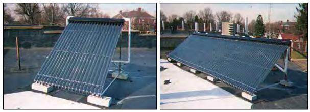
Figure A-105. Evacuated tube collectors installed on the EPA lab in New Jersey.
