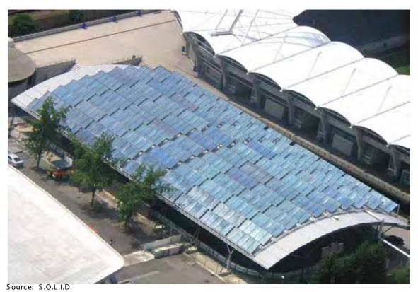
Figure A-17. Overview of the solar supported district heating network UPC arena Graz-Liebenau. The solar plant is operated on a "sale of energy" basis in cooperation with the company nahwaerme.at Energiecontracting GmbH, which was responsible for the funding and the proper operation of the plant, while S.O.L.I.D. was in charge of the design, planning, and erection.
