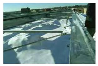
Figure A-96. Steel bracing.
