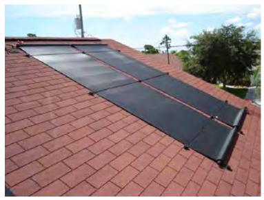
Figure 3.12. An unglazed solar mat-type solar collector made by FAFCO installed on a roof in California.
