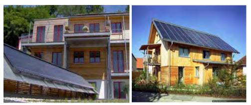
Figure 2.11. Two examples of aesthetic placements of collectors. At the right the collectors are integrated into the roof cover together with PV collectors at either side.
