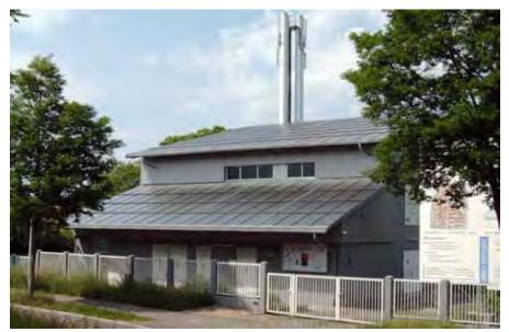
Figure A-63. Front view of the heating central with two roof-integrated collector areas.
