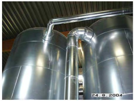
Figure A-64. Solar storage tanks.
