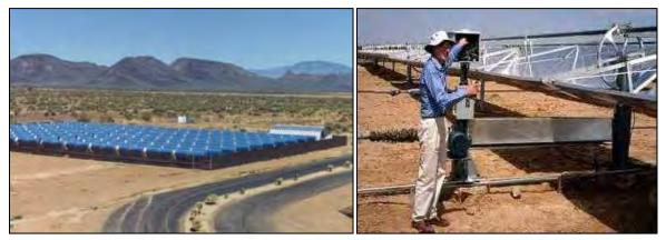
Figure A-125. Solar field of collectors at the Phoenix correctional facility (left); close-up of a row of parabolic collectors at the prison (right).
