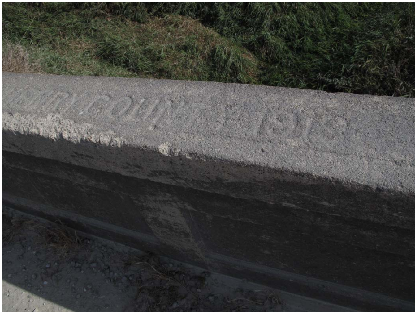
Photograph 44-02143-002 - Bridge, showing 1919 date stamp (October 2015)
