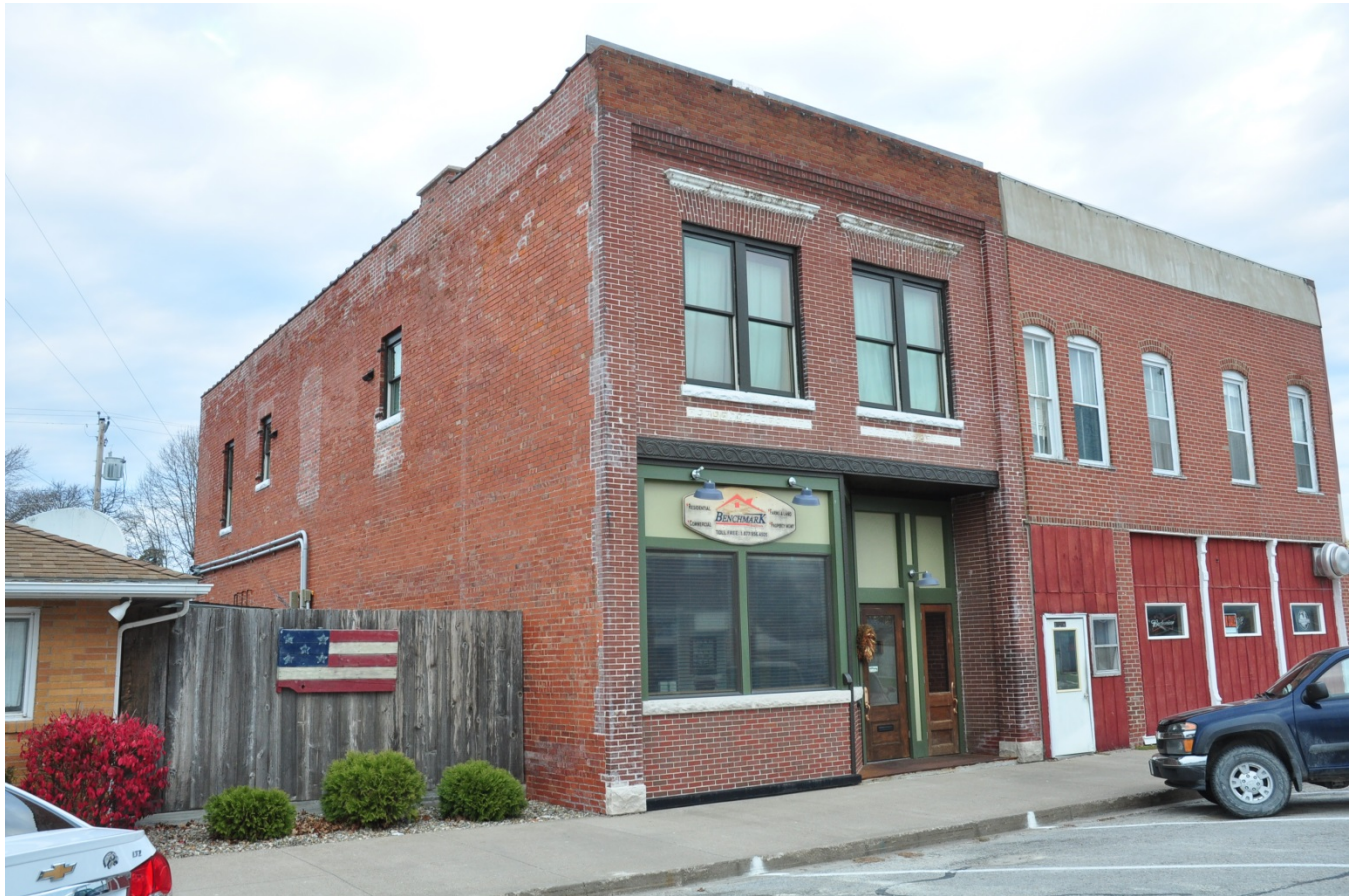
Photograph 44-01723-001 - Building, looking northeast (December 2015)
