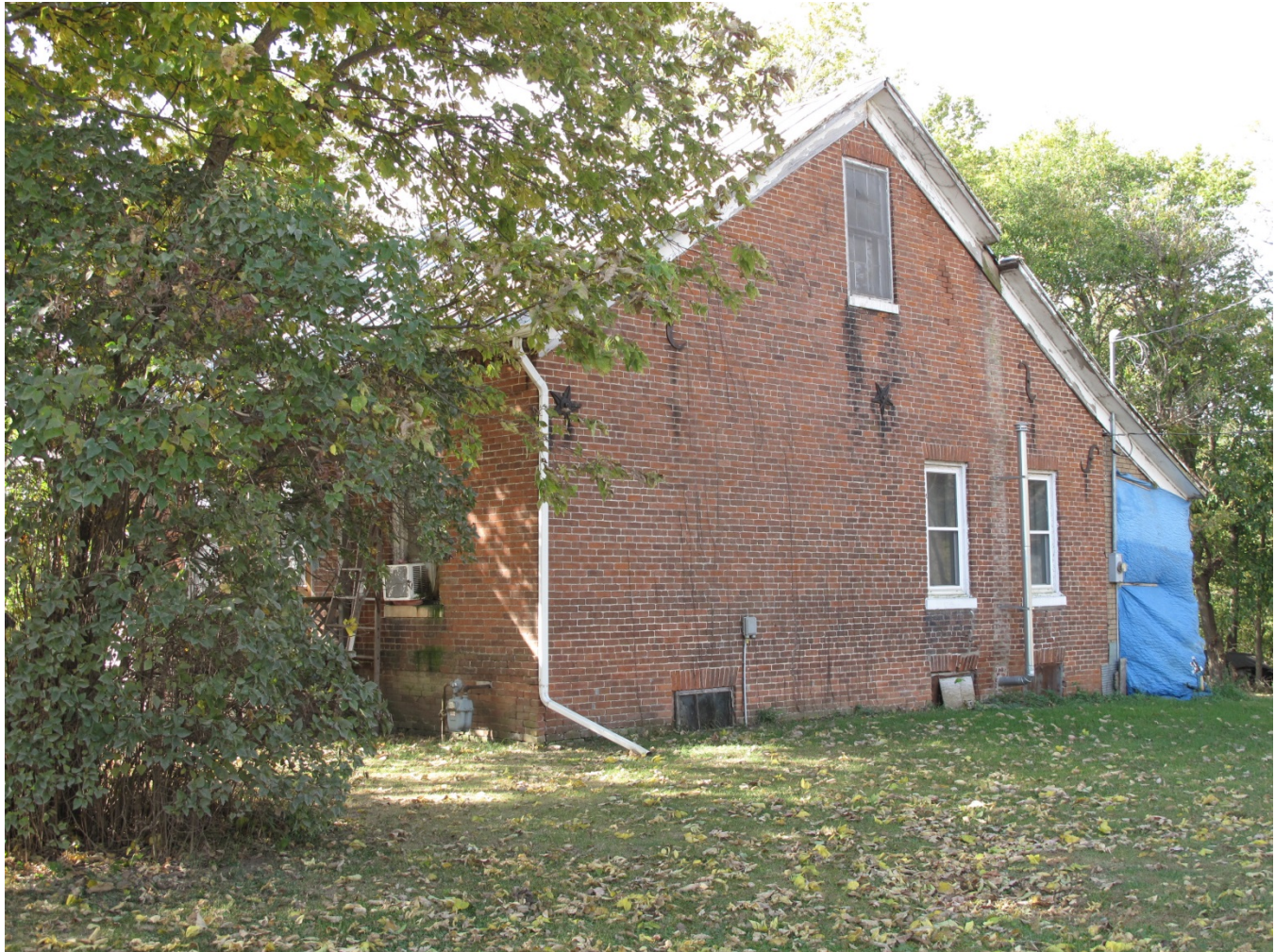
Photograph 44-02142-003 - House, looking southwest (October 2015)
