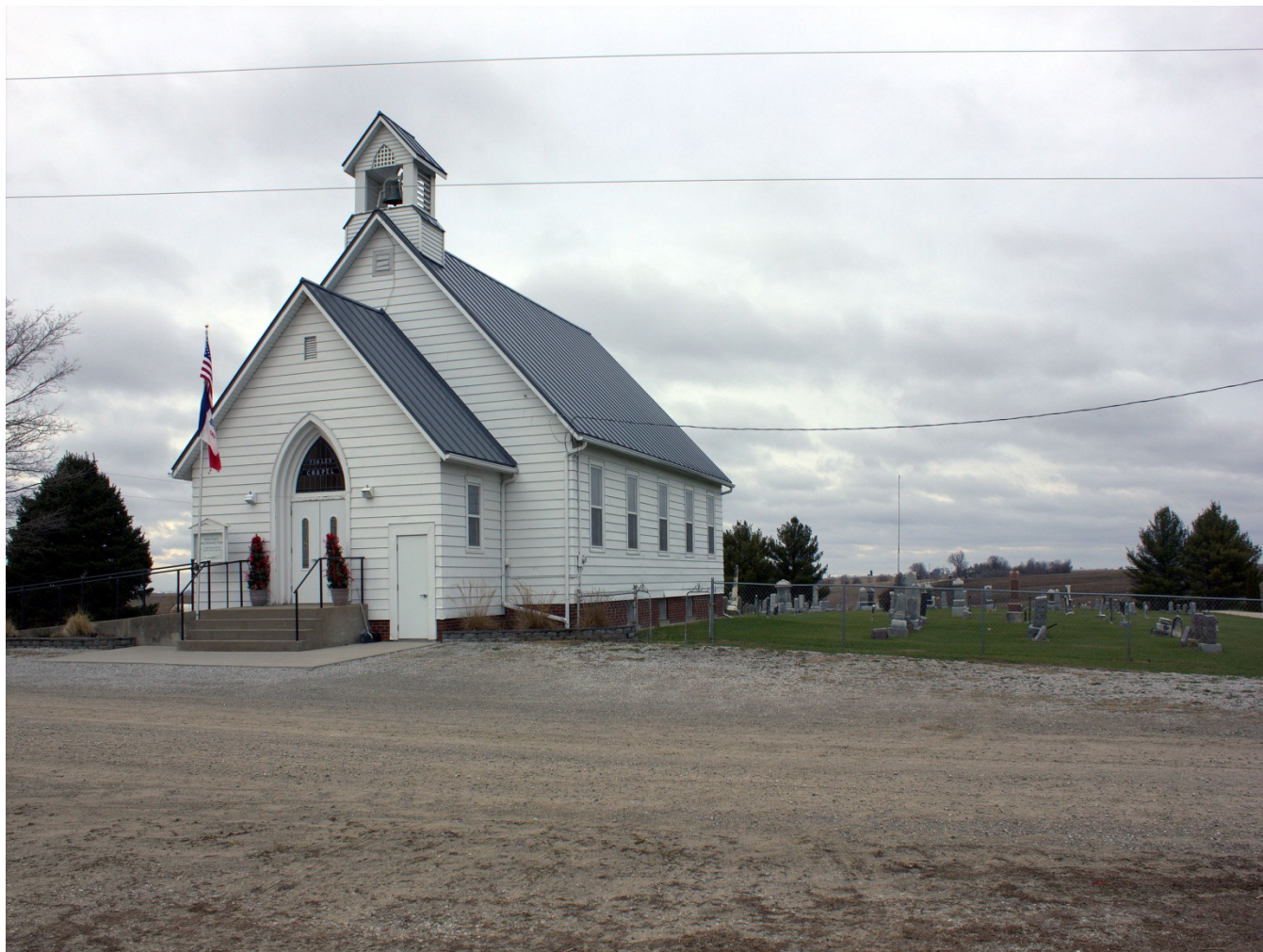
Photograph 44-02081-002 – Finley Chapel, looking northwest (December 2015)
