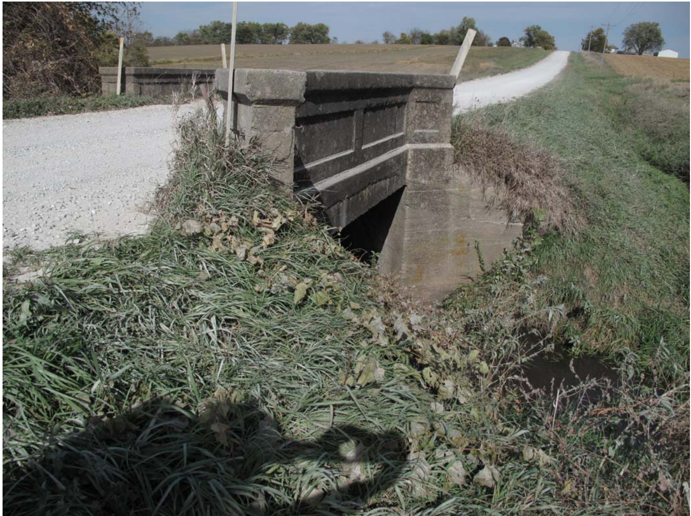
Photograph 44-02143-003 - Bridge, looking northwest (October 2015)
