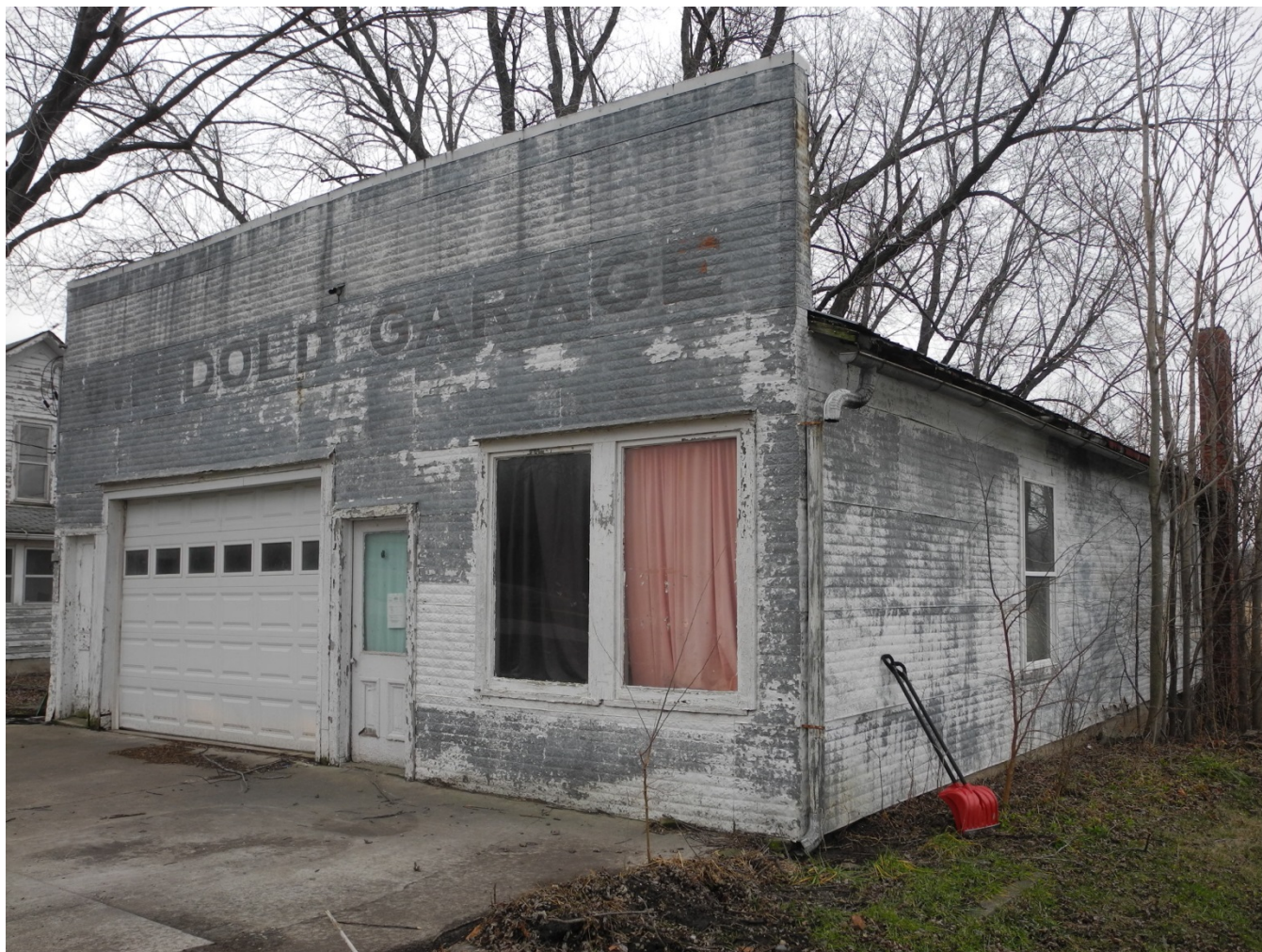
Photograph 44-02112-001 - Building, looking northeast (December 2015)
