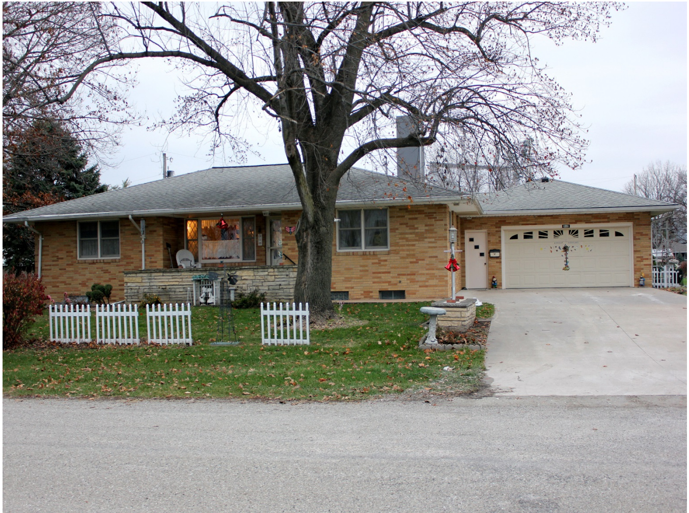
Photograph 44-01844-001 - House, looking north (December 2015)
