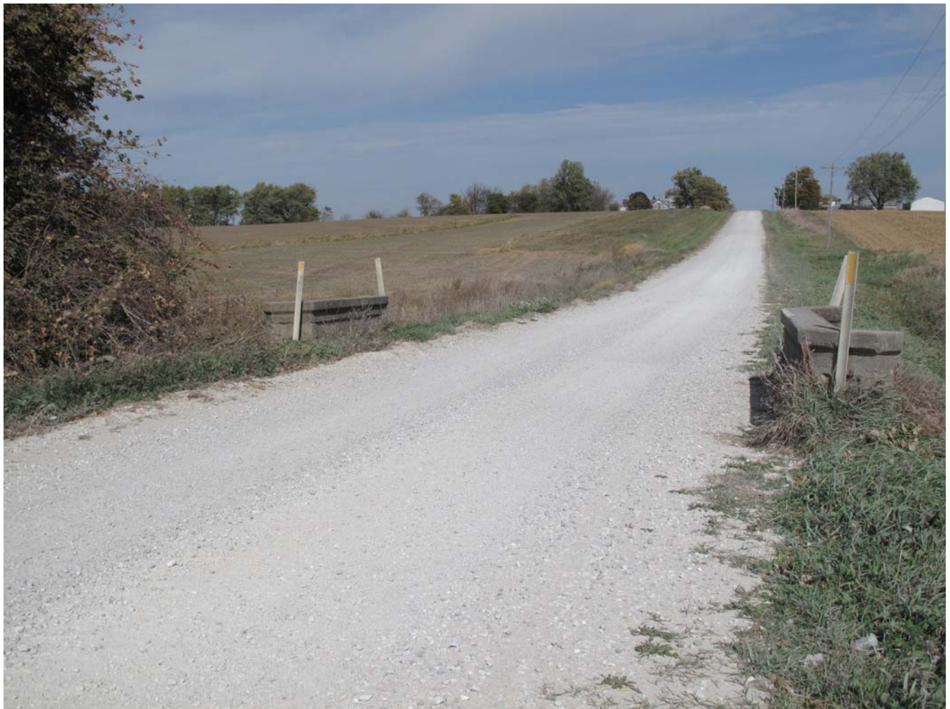
Photograph 44-02143-001 - Bridge, looking north on Gabriel Ave (October 2015)
