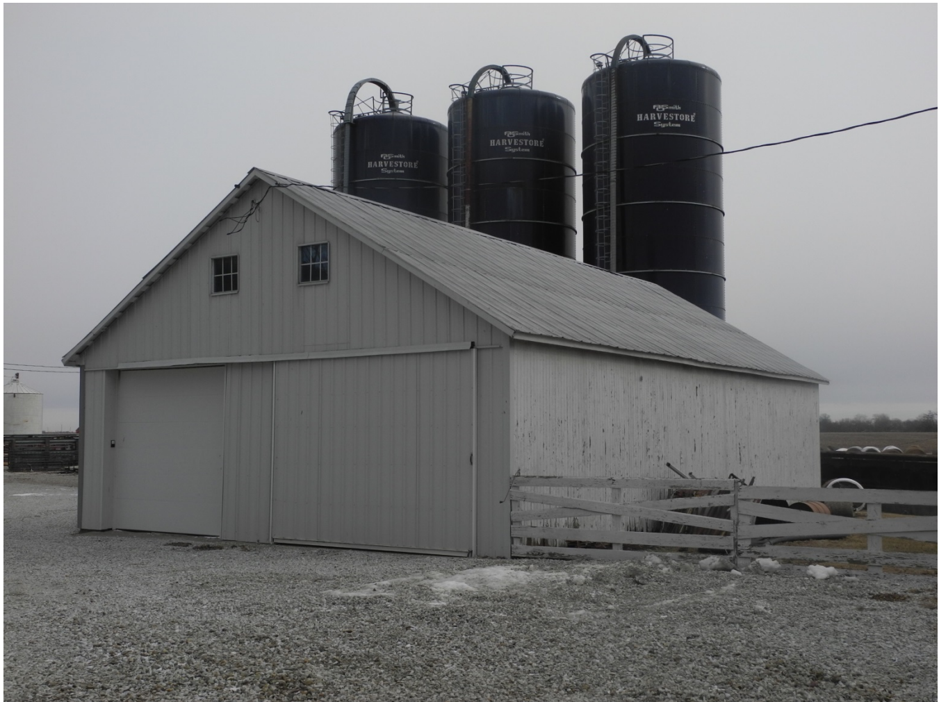
Photograph 44-02102-004 - Buildings, looking northeast (December 2015)
