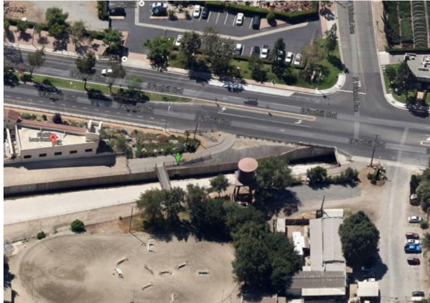
MTD 766 Aerial View
