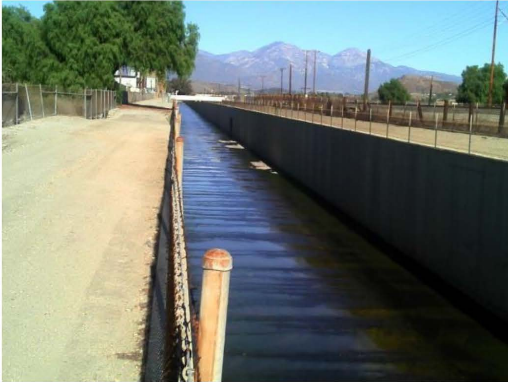
Figure 2-5. San Jose Creek TMDL site ESGV_SJC_DS Looking Upstream
