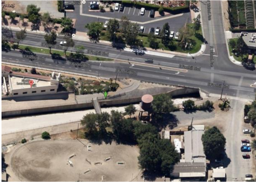
MTD 766 Aerial View
