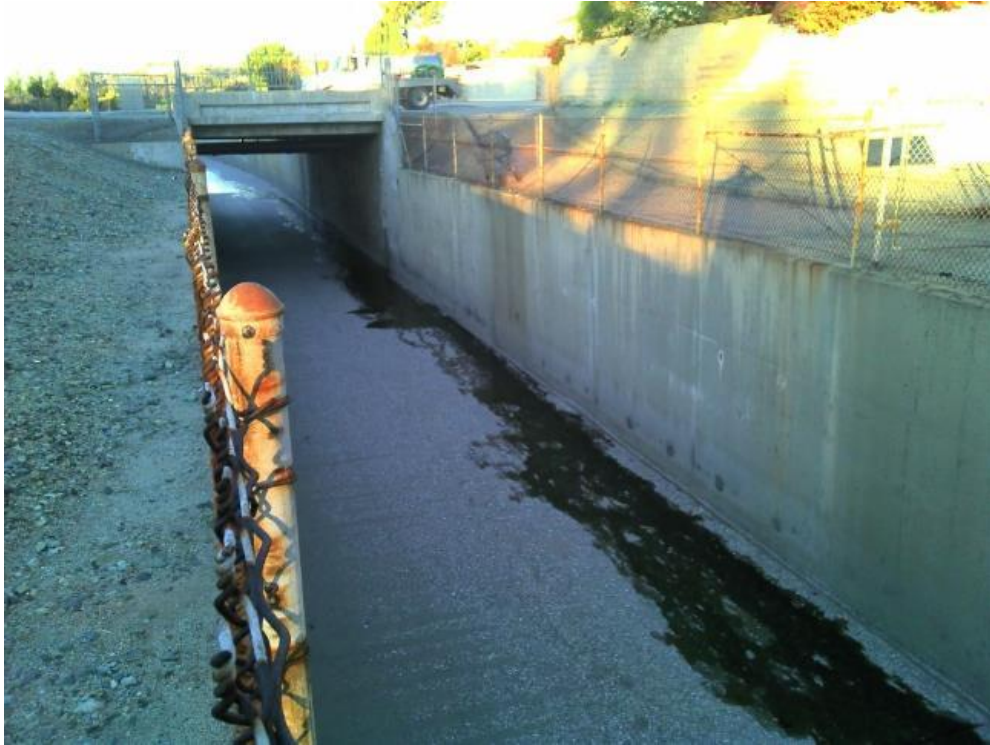
Figure 2-6. San Dimas Wash TMDL Site, ESGV_SDW_DS, Looking Downstream
