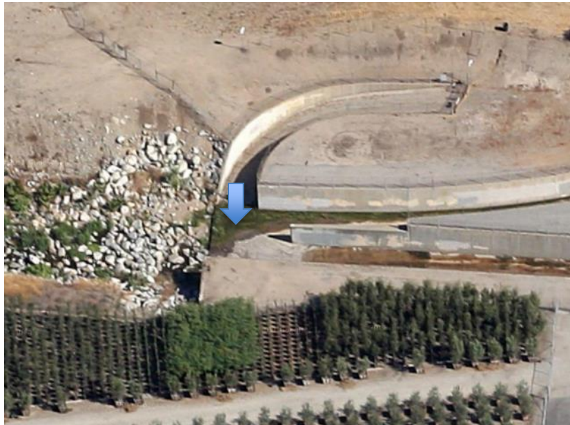
Figure 2-4. Confluence of Channels Discharging to Puddingstone Reservoir at Transition Between Hard and Soft Bottom Channel.
