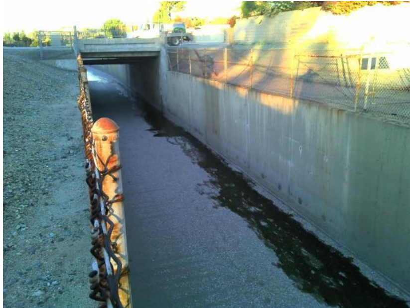
ESGV_SDW_DS Looking Downstream
