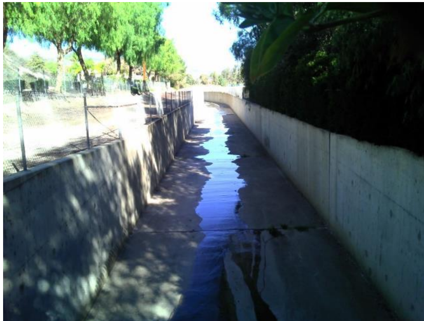
ESGV_LOW_DS Puddingstone Channel Flow Monitoring Location Looking Upstream
