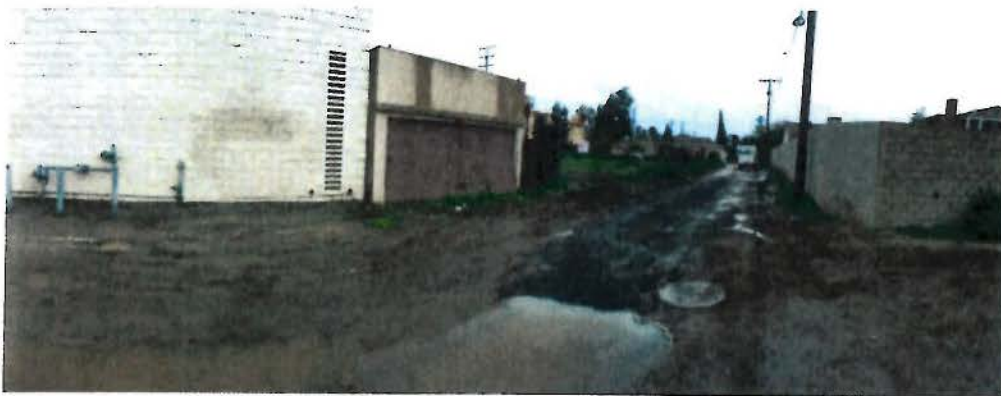
Figure 2. Existing conditions of the alley.
