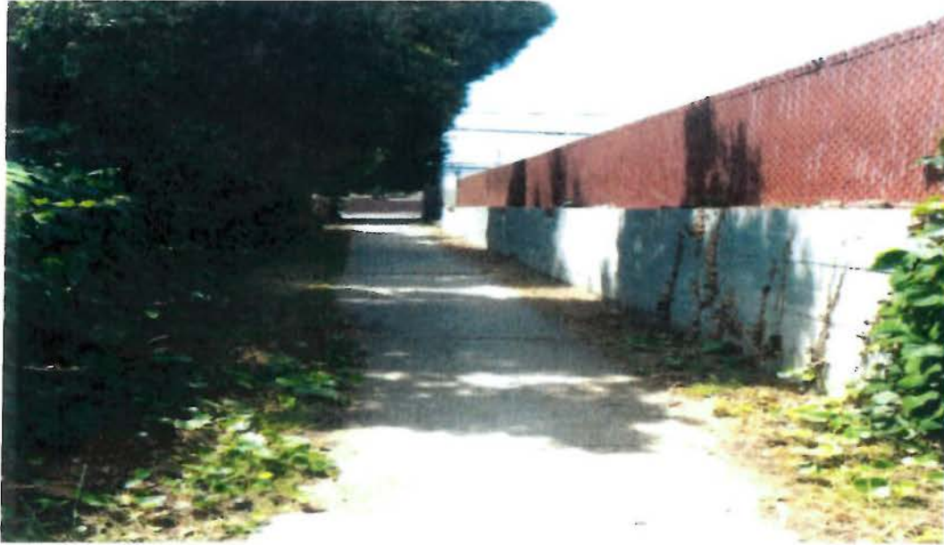
Figure 8A: Pedestrian alley from West Manchester Avenue
