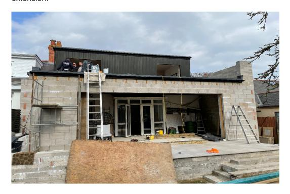
10. During the investigation, it was also identified that the rear extension was being built onto and tied into the external wall of a neighbouring property, with
